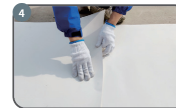
Self-adhesive Overlap or HotAir Welding
