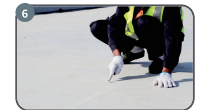
Inspection and Acceptance
