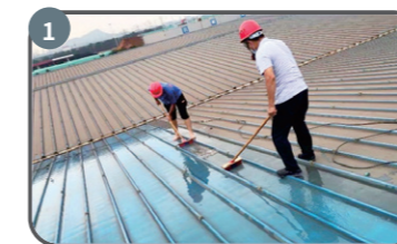
Cleaning and Derusting of Original Roof Color Steel Sheet
