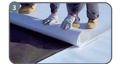
Paving the Membrane while Uncovering the Bottom Isolation Film
